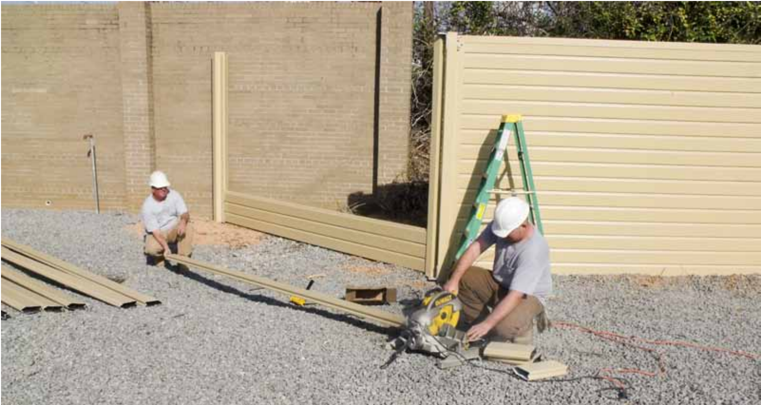
Carsonite sound barrier planks are adjustable and can be cut in the field.
